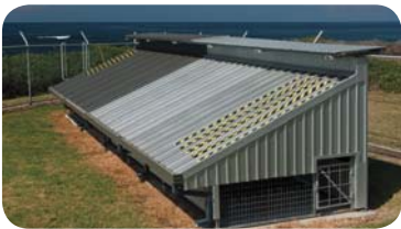
Purpose built test structure made from next generation ZINCALUME® steel AM125 exposed to four years of extreme conditions less than 100m from breaking surf, Bellambi NSW.
